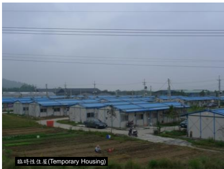
臨時性住屋(Temporary Housing)
